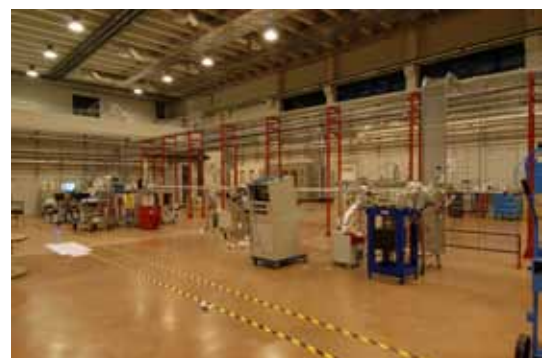
Experimental hall at FERMI, February 2011. The FERMI crew has started to install the first beamline.
